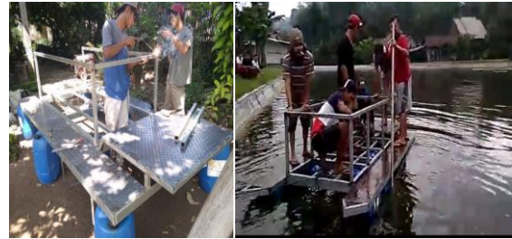
Figure 2. Construction of garbage scaffolding and sediment boats in reservoirs
